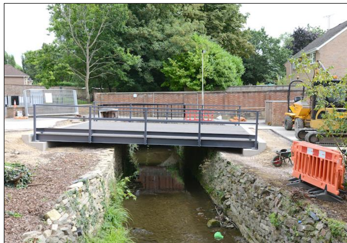
Figure 3.1: Example of temporary span bridge
